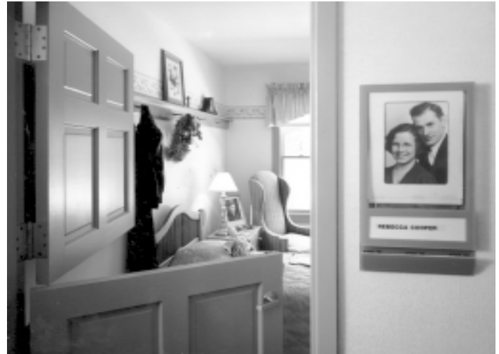
Dutch doors allow for privacy, yet provide residents at Woodside Place with the ability to look into the rooms. Perkins Eastman Architects
