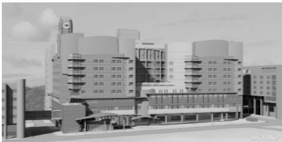
Interpreting themes of healing in materials, shape and color is the philosophy behind the design of the new Children's Hospital of Pittsburgh. Designed by Astorino.
